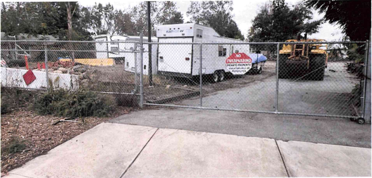
The existing chain-link gate and perimeter fencing along the 17th Street frontage of the project site
