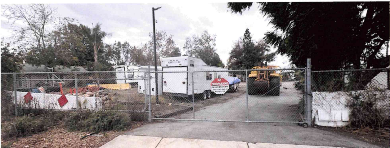
View looking North from 17 th Street. Site Inspection November 20, 2025.
